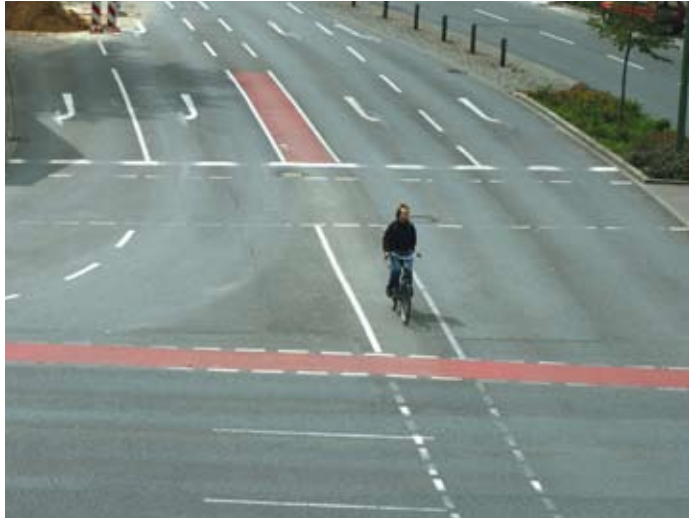
Figure 29. Dashed bike lane provides guidance through a wide intersection in Osnabrück, Germany. 6
