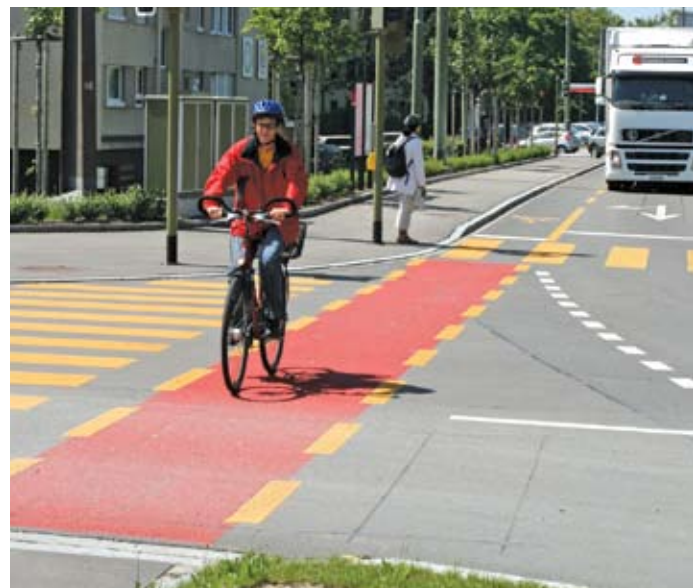
Figure 28. Colored bike lane at potential conflict area in Winterthur, Switzerland.
