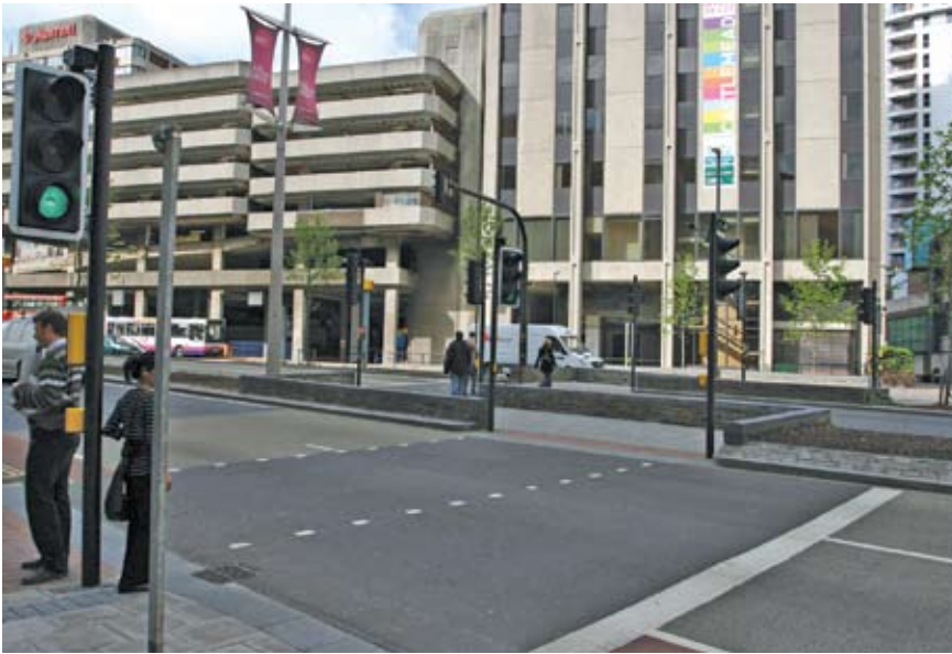
Figure 12. Offset pedestrian crossing at a signalized intersection in Bristol, United Kingdom.
