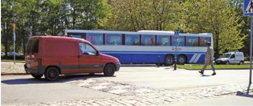
Figure 14. Raised crosswalk at two-lane roundabout exit in Malmö, Sweden.
