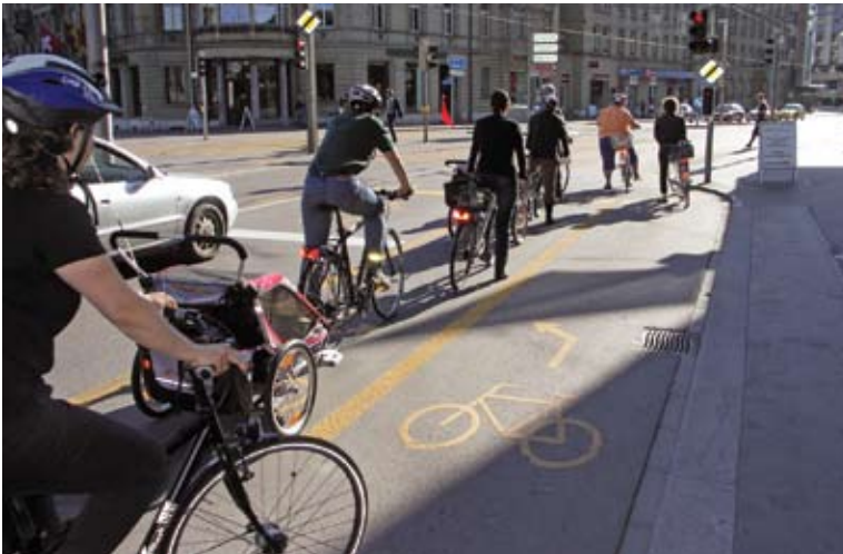
Figure 24. Advance stop lines for onstreet through and left-turn bike lanes in Bern, Switzerland.
