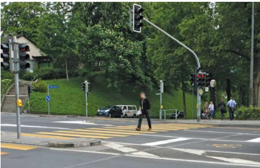
Figure 13. Near-side traffic signals in Bern, Switzerland.
