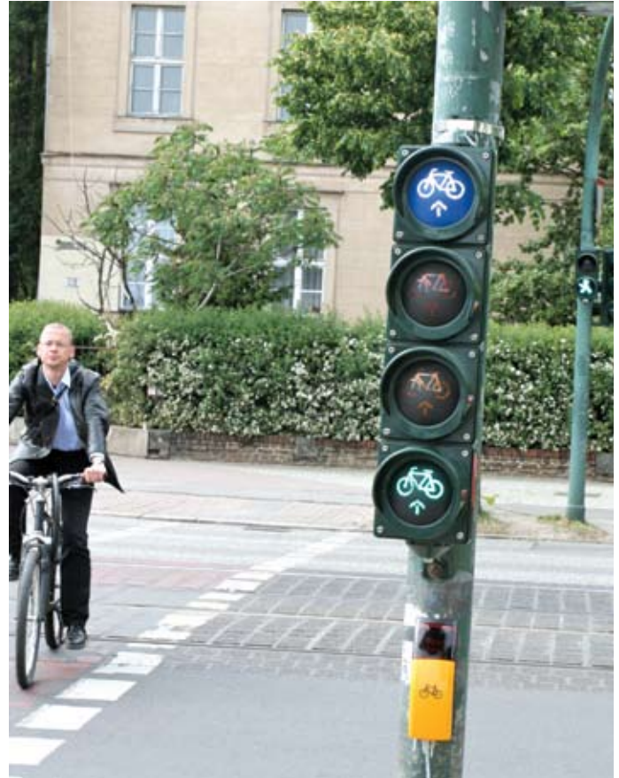
Figure 27. Bicycle traffic signals control bicycle traffic movements at signalized intersections in Potsdam, Germany. (Note: A blue plaque placed in the highest signal lens is not intended to control bicycle movements.)
