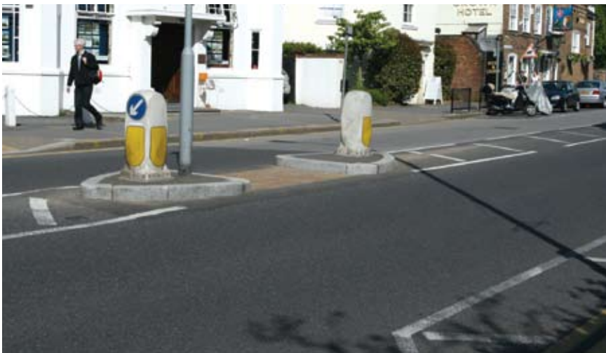
Figure 15. Median island with unmarked crosswalk in London, United Kingdom.
